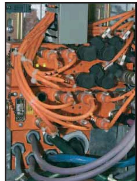
PROFIBUS modules with M23 or M12 connections.
